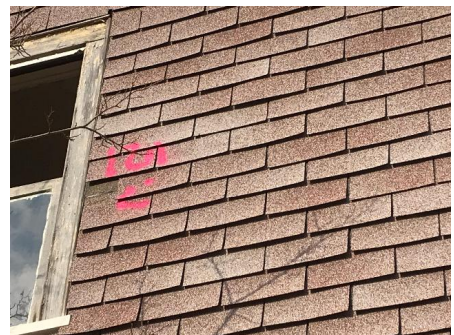
Sample ID: AS 12-2 Notes: Red Square Asphalt Siding
