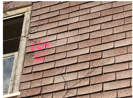
Sample ID: AS 12-1 Notes: Red Square Asphalt Siding
