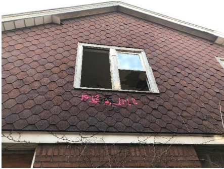
Sample ID: AS 10-1 Notes: Red Octagonal Asphalt Siding
