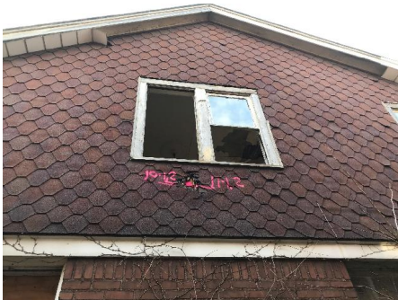
Sample ID: AS 10-2 Notes: Red Octagonal Asphalt Siding
